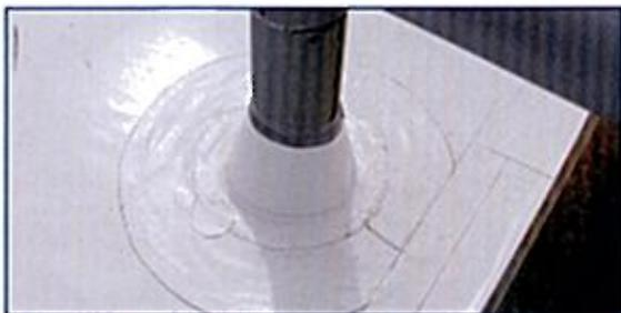
All rooftop penetrations are heat-welded by hand to provide complete watertight application.
