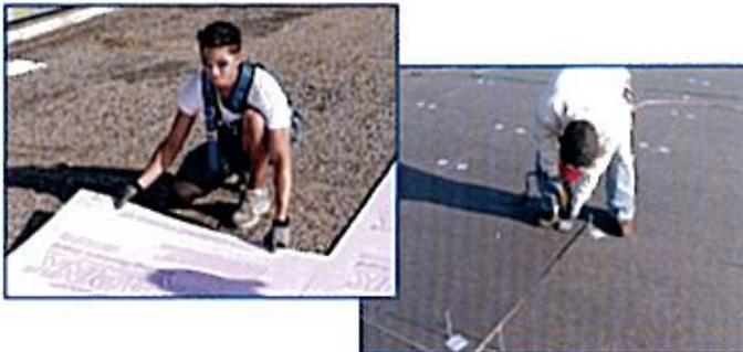
Insulation is mechanically fastened and installed over the existing roof.
