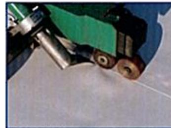
Seams are heat welded to provide the strongest seam of all single ply membranes.
