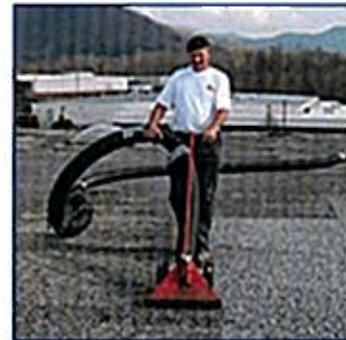
Preparation of the roof by vacuuming loose gravel.
