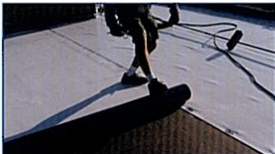
Membrane is rolled into place and then installed by mechanically fastening, adhering or ballasting.
